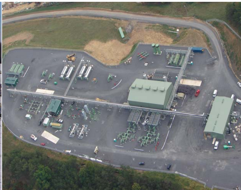
Transmission and Storage Compressor Station Columbia Gas Transmission Baker, WV
