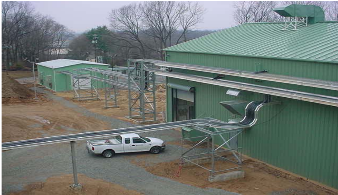
Transmission Compressor Station Columbia Gas Transmission Downingtown, PA
