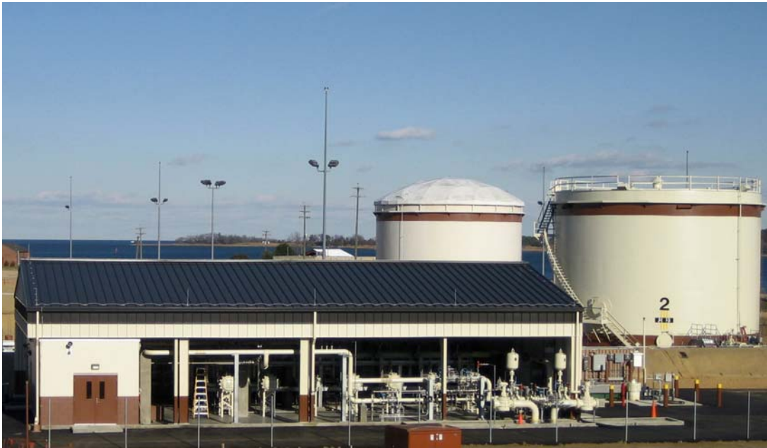
Replace Hydrant Fuel System Langley AFB Hampton, VA
